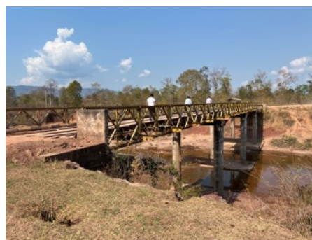
Picture 28 Concrete substructure of the major steel bridge.
