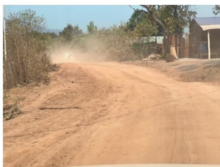
Picture 25 Lack of drainage in several sections of road 7271
