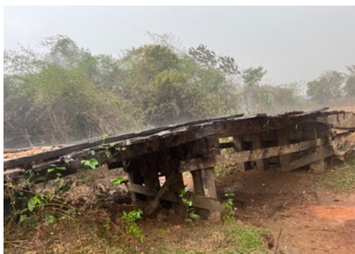
Picture 37 Community built bridges in areas prone to flooding.
