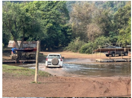
Picture 34 Bridge required to make this road accessible.
