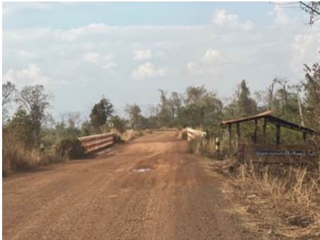
Picture 19 Concrete bridge on 6909
