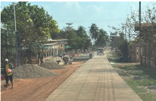
Picture 1 Community funded concrete cement pavement
